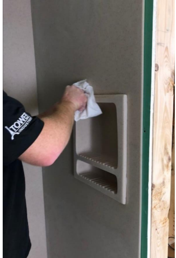
Wipe Away Adhesive around Holder (Step 6)
