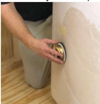
Drain Assembly at base (Step 7)
