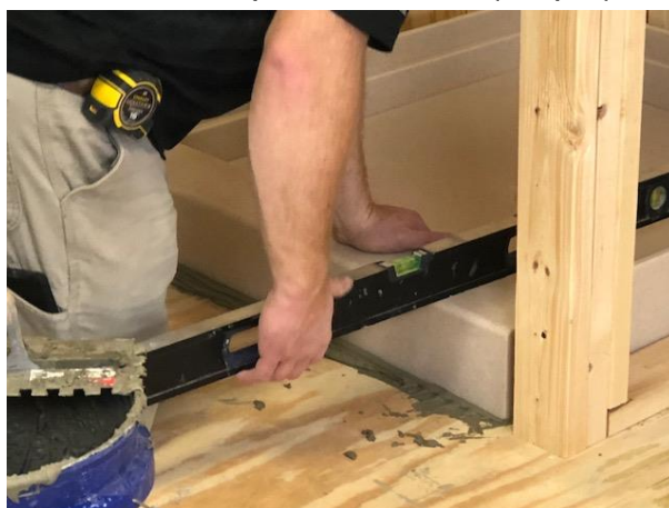
Level on top of Threshold (Step 9)
