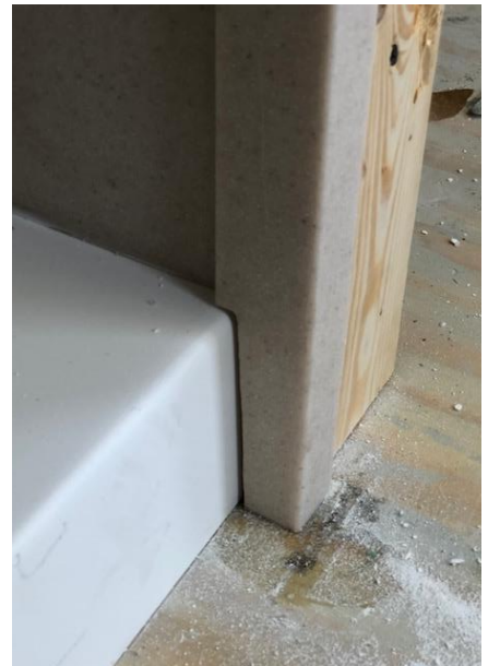
Outside Corner Mold at Base
