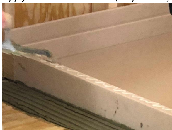
Apply Thinset and Sealant (Steps 5 & 7)
