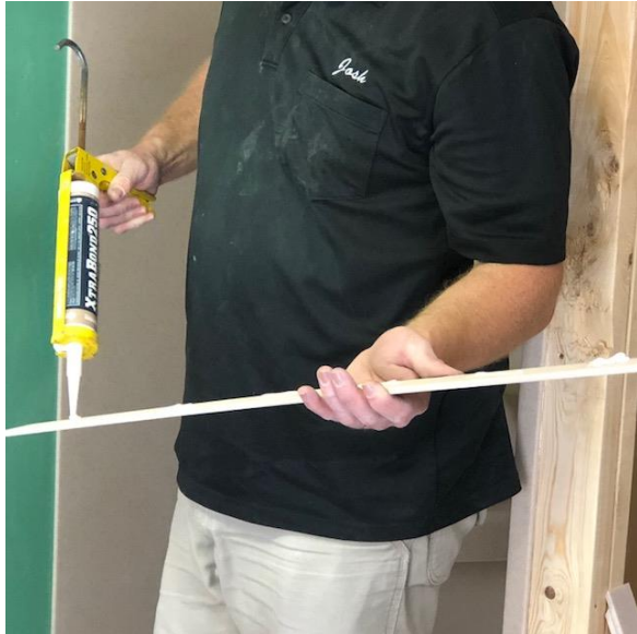
Apply adhesive to trim molding (Step 4)
