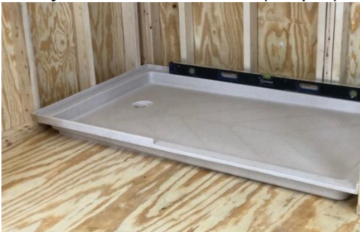
Dry Fit Base and Level (Step 4)
