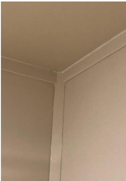
Batten at Inside Corner Mold
