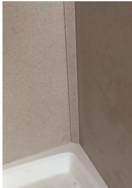
Inside Corner Mold at Base
