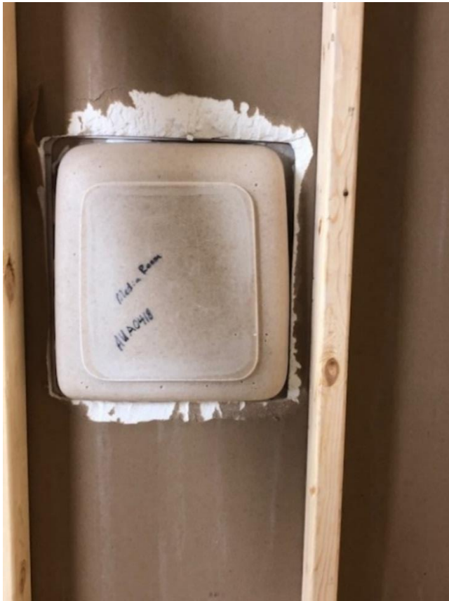
Back side of Recessed Holder in Wall (Step 6)
