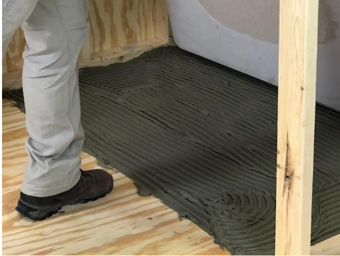
Apply Adhesive using 1/2" Notched Trowel (Step 8)
