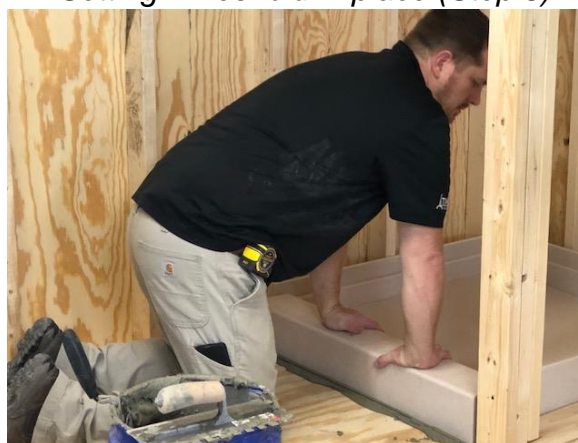
Setting Threshold in place (Step 8)
