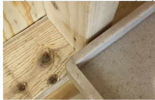
1/8" Gap between wall and base (Step 4)
