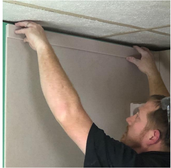
Install Batten at top of panel. (Step 5)
